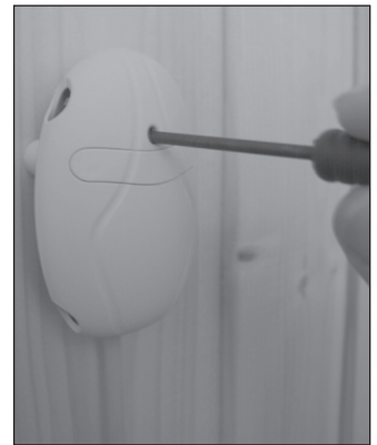
Figure 11. Reset button for overheating limiter
